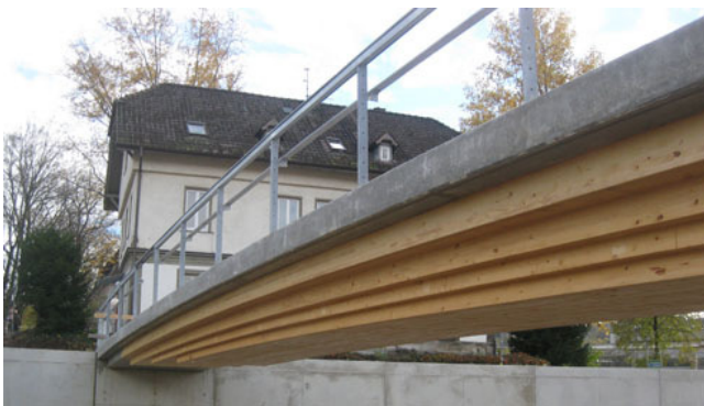
Fig.1: Composite timber-concrete foot bridge in Schwäbisch Gmünd, Germany [8].
