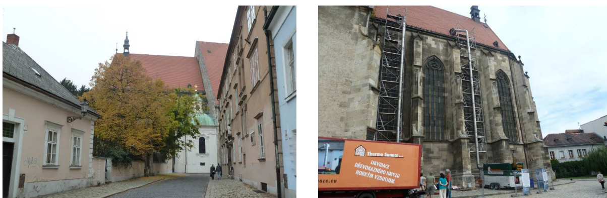
Fig. 1 The roof structure and the installation of the fumigator with the hot-air pipeline
