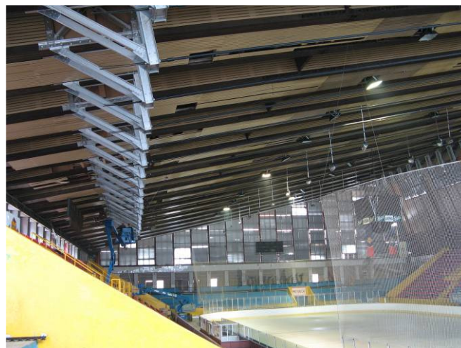
Fig. 11 View of the Reconstructed Roof Structure
