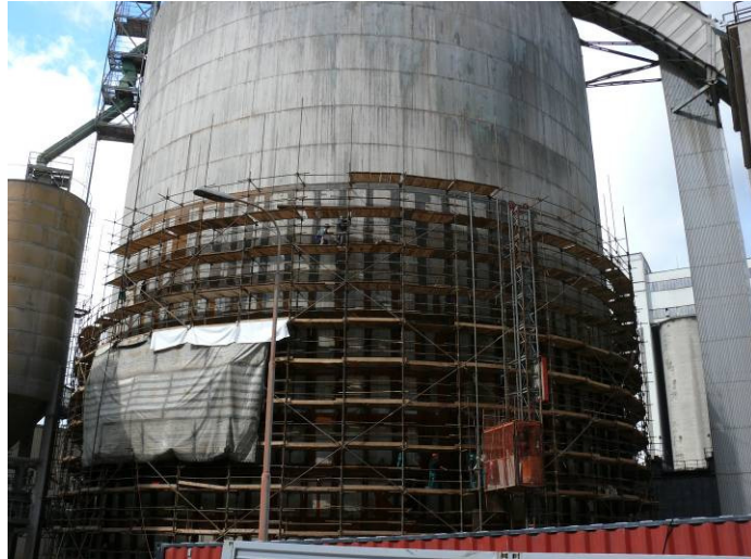
Fig. 8 Reconstruction Works on the Clinker Silo
