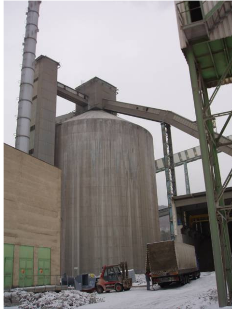
Fig. View of Clinker Silo PC2 with Technology
